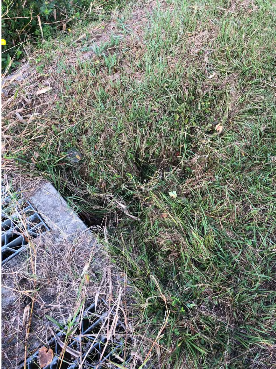
Site 18 Erosion in front of weir
